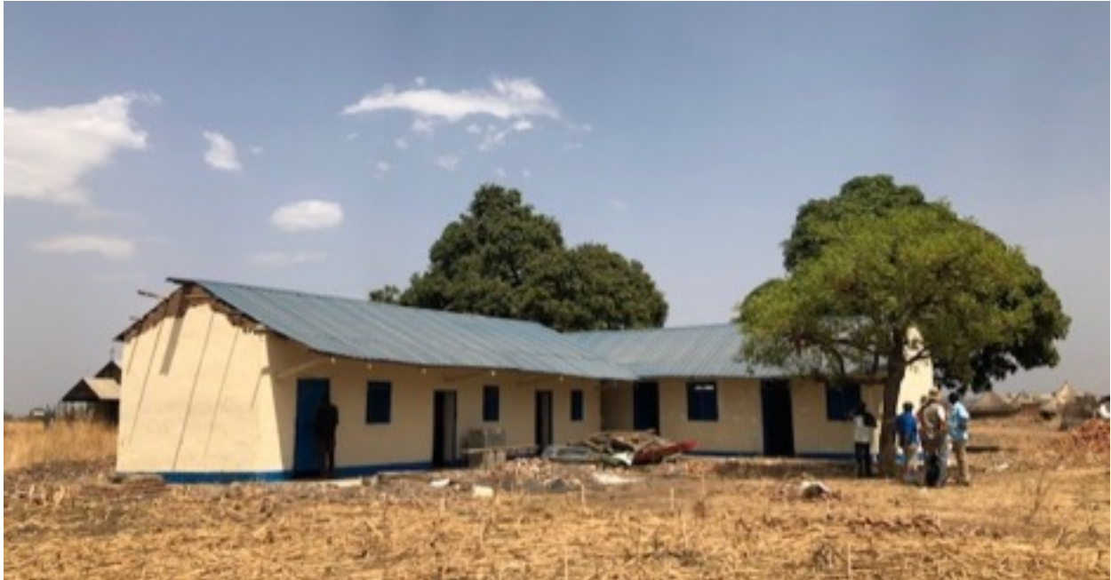
The new health clinic constructed on the East Bank with funds secured by HART from the Guernsey Overseas Aid and Development Committee
