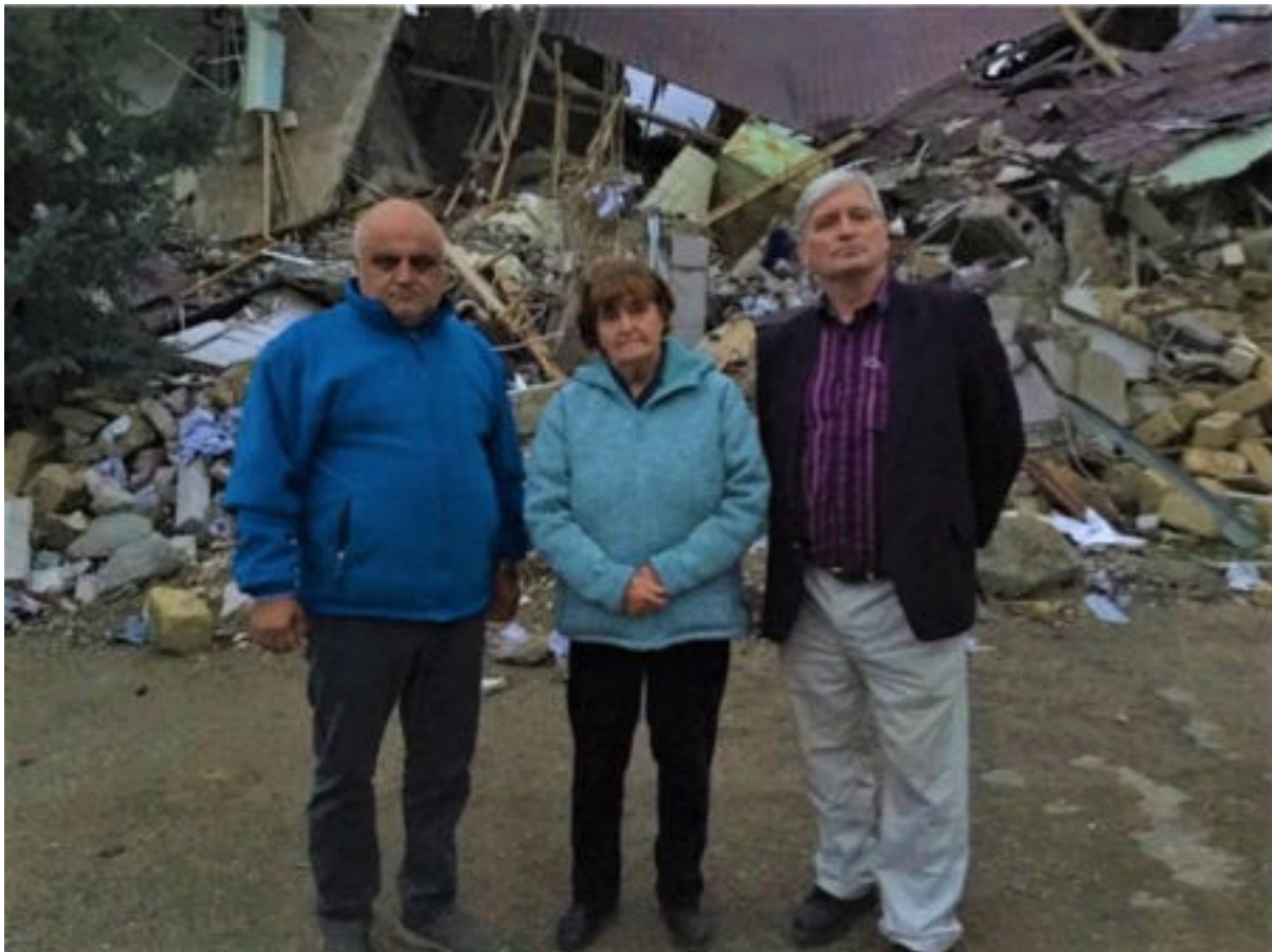
Vardan Tadevosyan, director of the Lady Cox Rehabilitation Centre in Nagorno Karabakh, with Caroline Cox and David Thomas surveying the damage to an electrical power station in Stepanakert.
