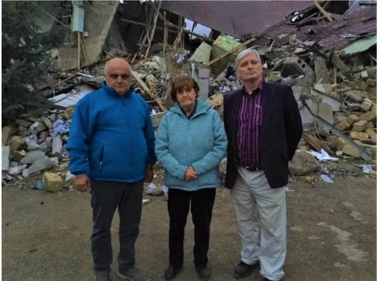
Vardan, Baroness Cox and David Thomas survey the damage to an electrical power station in Stepanakert. Civilians hiding in basements were without heat and light.
