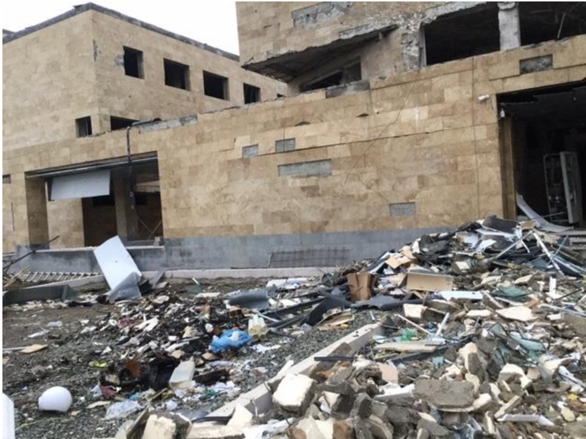
The aftermath of Azerbaijani bombing which targeted and destroyed this maternity hospital in Stepanakert.
