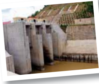
Above: The Shweli Hydropower Dam 1, located in Mantat village, northern Shan State
