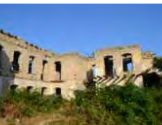
Above: A damaged building in Nagorno-Karabakh
